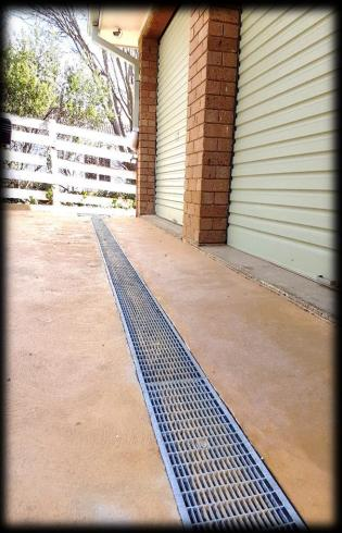
Bowral Denture clinic, was getting flooded when the weather turned grey. Since the SABDrain 601 150m x 150m has been installed the issue of flooding is a thing of the past.
